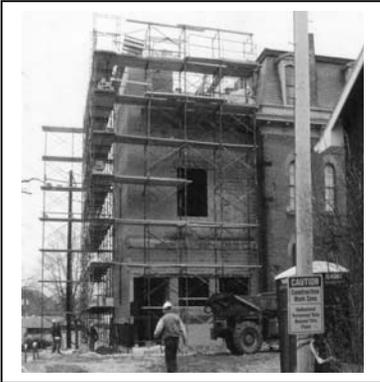
Our building addition to make the Town Hall Museum accessible to everyone is about 60% completed at this date. The outside of the structure is up and workers have been busy inside installing plumbing, lighting, dry wall and, of
